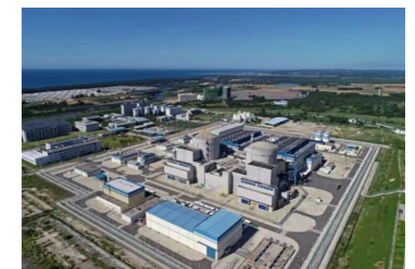
Hainan Changjiang Nuclear Power Plant
